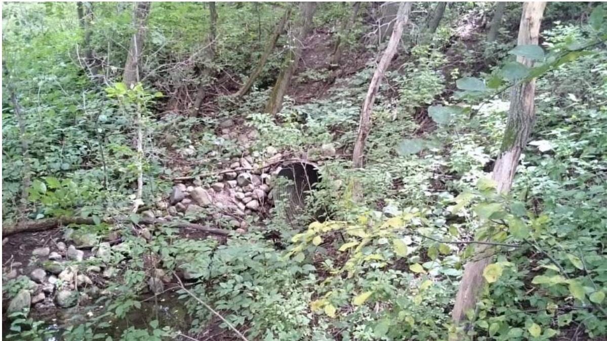
Photograph 1 is facing south looking at the outlet culvert.
