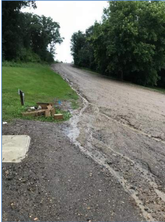
Photograph 12 is looking uphill at Huggett Lane from the intersection of Webster Boulevard. This is an example of where the secondary ditches in the road need to be repaired (Dan Pearson - 2019).
